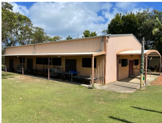
Current Performing Arts Centre. Opened in 2003 with community funding. Shed structure.
